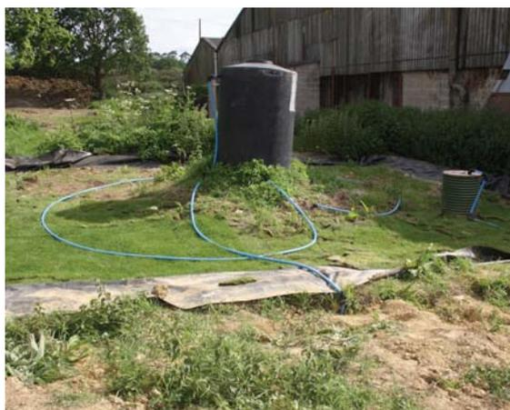
Lined biobeds can treat sprayer washings and drainage from pesticide handling areas
